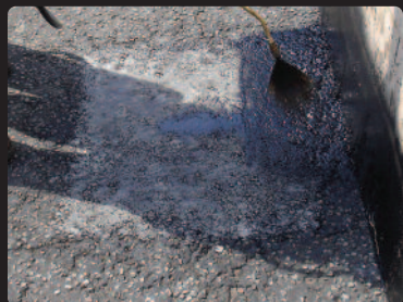
➤ Applying Rhinophalt® preservative
