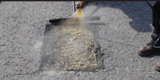
➤ Applying Rhinobinder® rejuvenator
