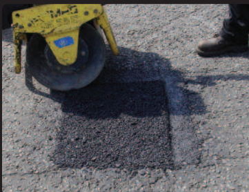
➤ Compaction of repair
