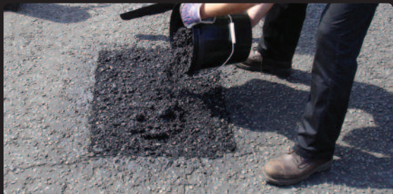
➤ Adding cold replacement material
