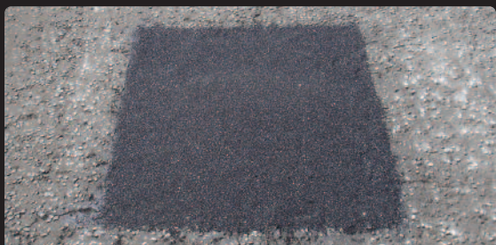
➤ Permanent Rhinopatch® repair, completed in only 15 minutes
