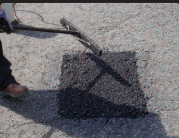
➤ Levelling of materials
